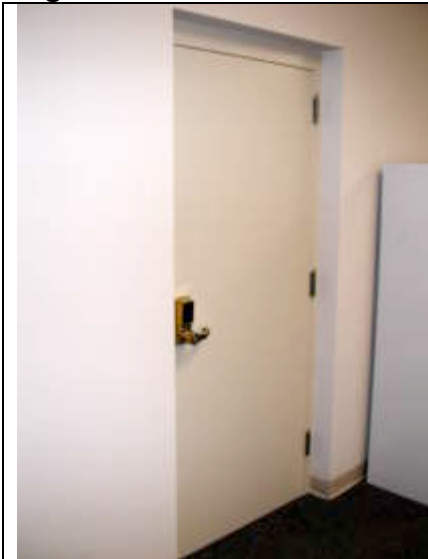
Figure 3.3 Server Room Entrance
