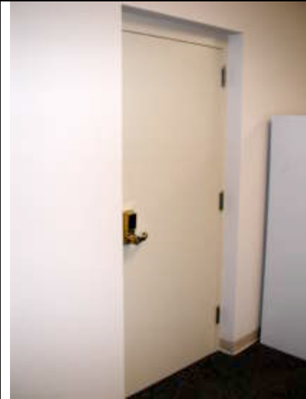
Figure 3.3 Server Room Entrance
